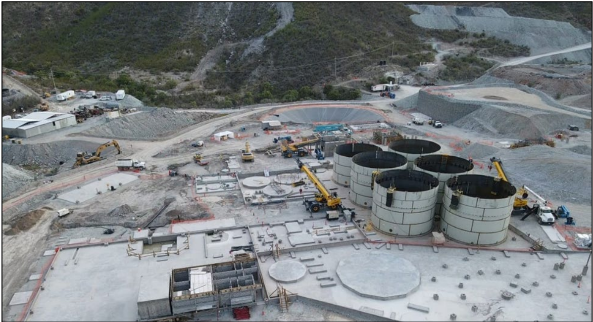
Figure 4: Leach Tank Construction
