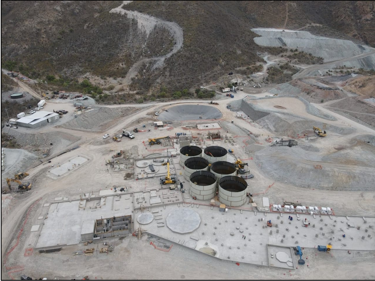
Figure 3: Overview of Process Plant Area
