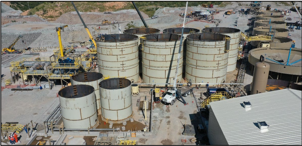
Figure 4: Leach Tank Construction
