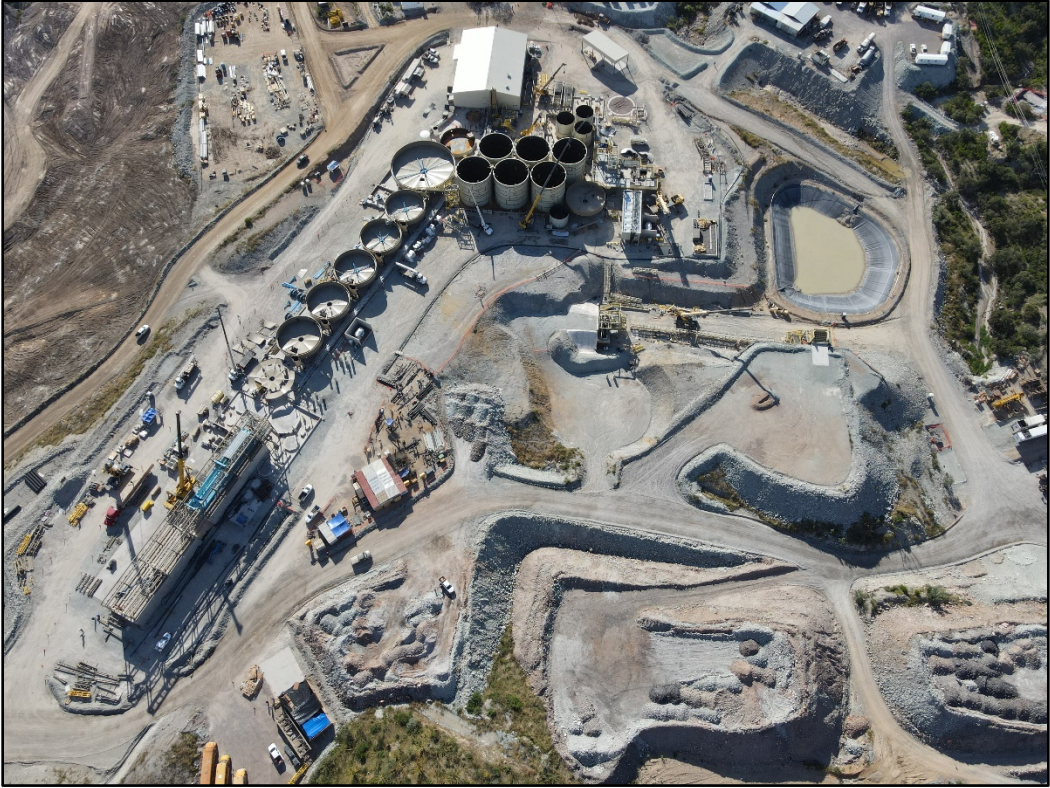
Figure 1: Drone Image of Process Plant Construction and Stockpiles
