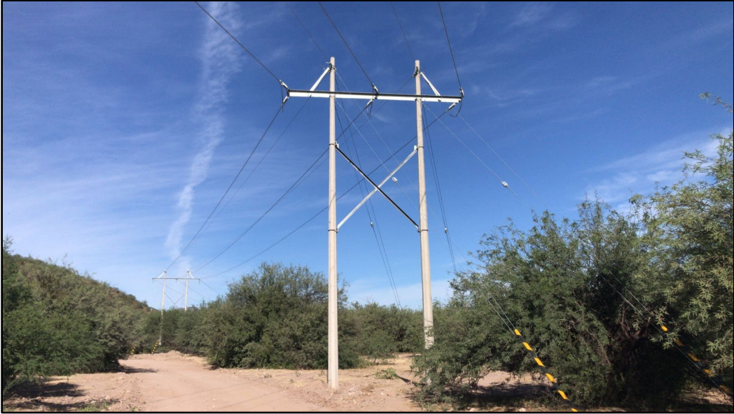
Figure 5: Powerline Pole Installation
