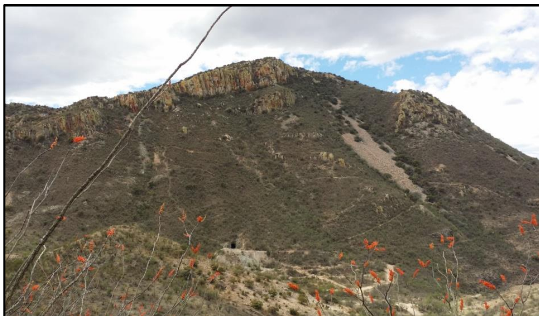
Photo 6-9: View of Babicanora Central Portal and Site of Historical Processing Facility, November 2017
